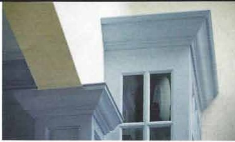
Well-designed crown molding details of the kitchen cabinetry add a finished touch.
